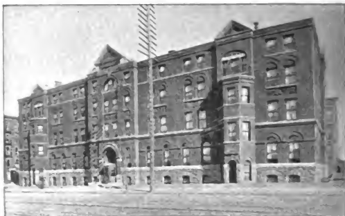
METHODIST EPISCOPAL CHURCH HOME, AMSTERDAM AVENUE AND WEST 93D STREET.
